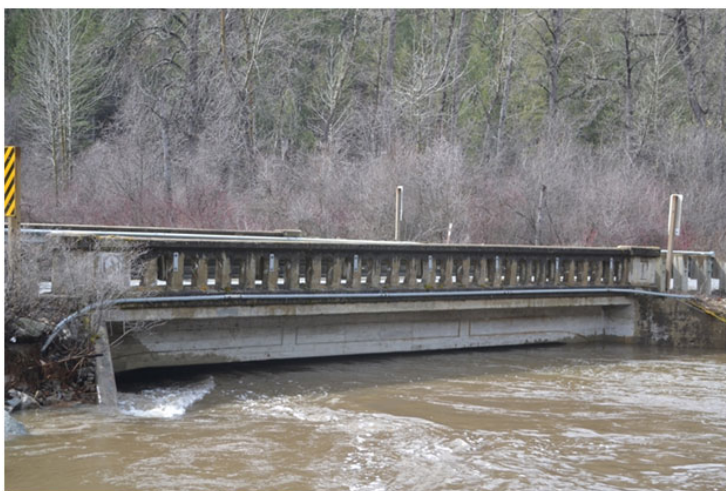
State Highway 21 Bridge at 25 mile, April 10 2017
